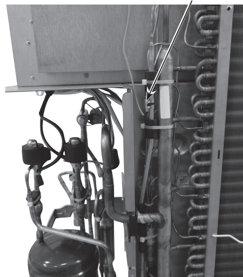
Thermistor <Liquid> (TH3)
